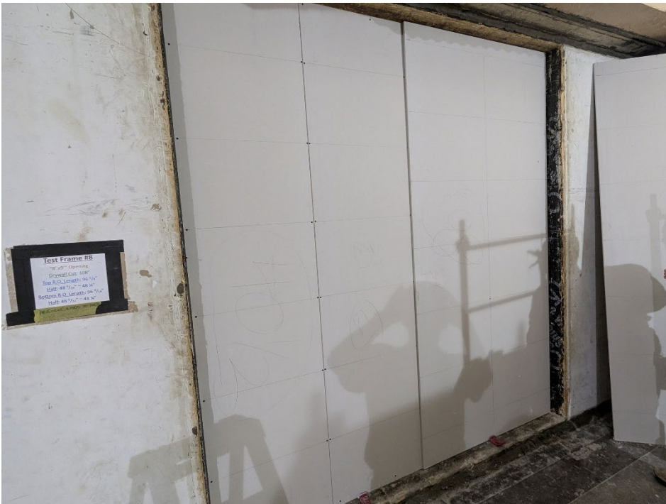
Figure 10 – Face layer gypsum partially installed on receive room side
