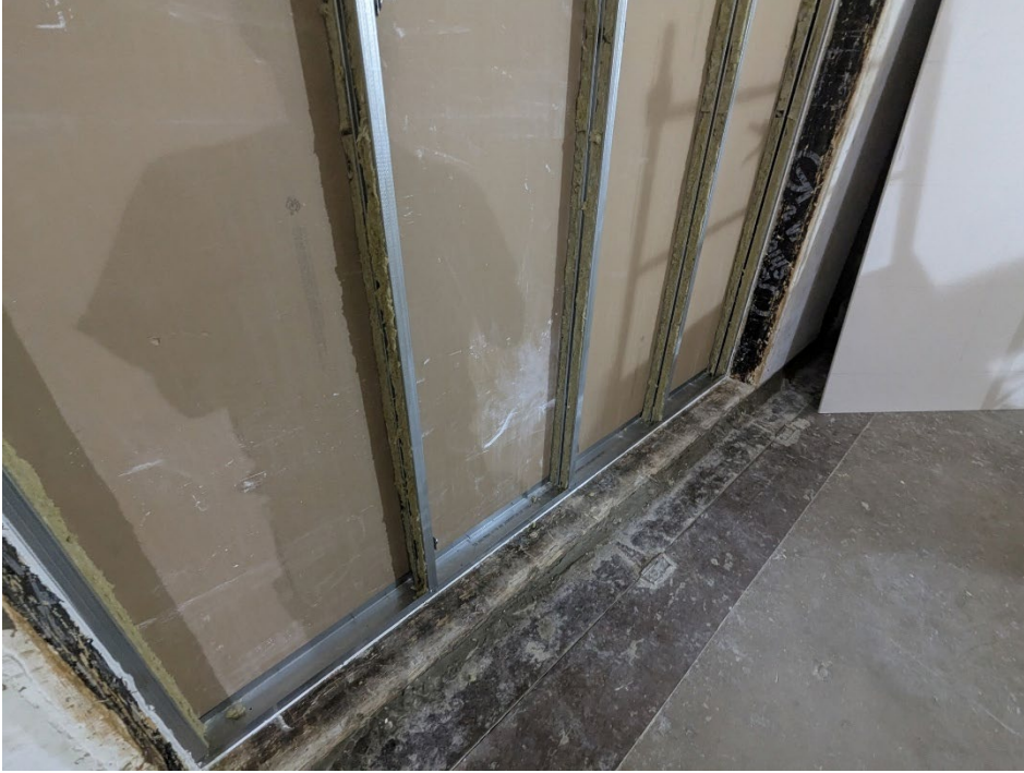
Figure 7 – Insulation installed inside studs, viewed from receive room
