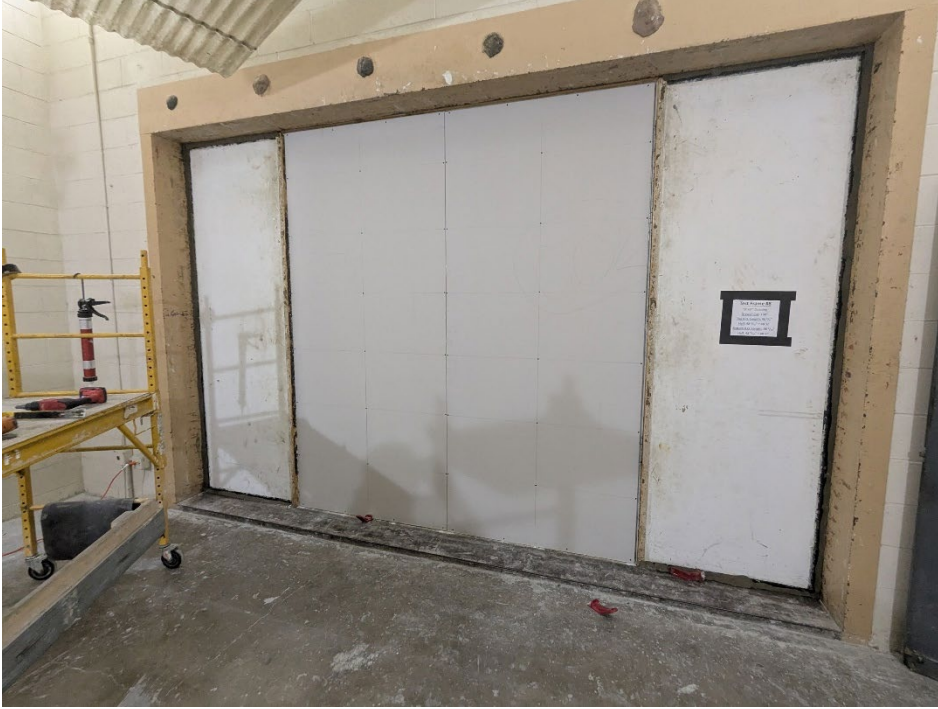
Figure 5 – Base layer gypsum board installed on source room side
