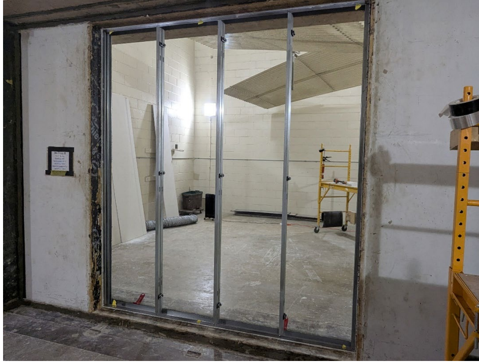
Figure 3 – Tracks, studs, and clips installed in test aperture
