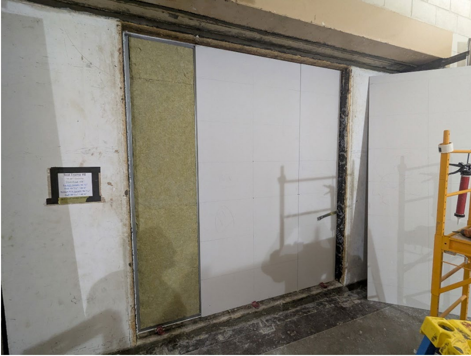
Figure 9 – Base layer gypsum partially installed on receive room side
