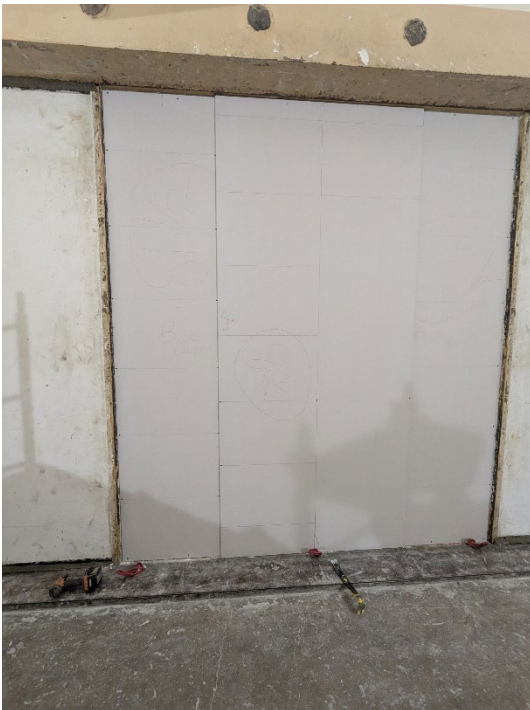
Figure 6 – Face layer gypsum board partially installed on source room side
