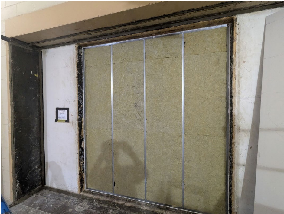
Figure 8 – Insulation installed in stud cavities
