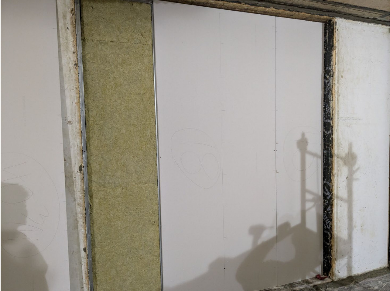
Figure 7 – Gypsum partially installed on receive room side
