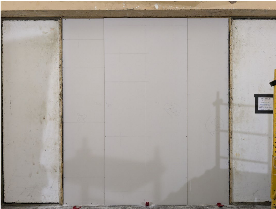
Figure 6 – Face layer gypsum board partially installed on source side
