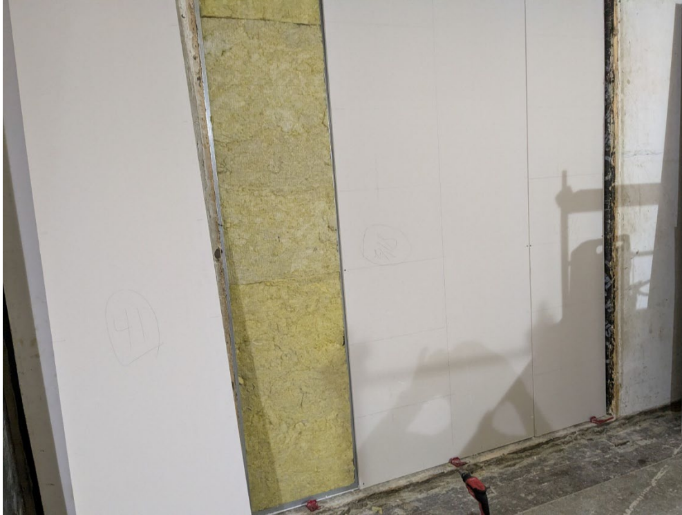
Figure 9 – Base layer gypsum board partially installed on receive side
