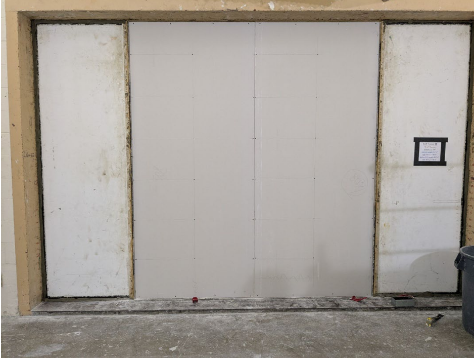
Figure 5 – Base layer gypsum board installed on source side
