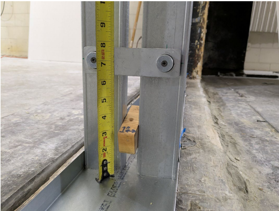
Figure 4 – Detail of studs and clips
