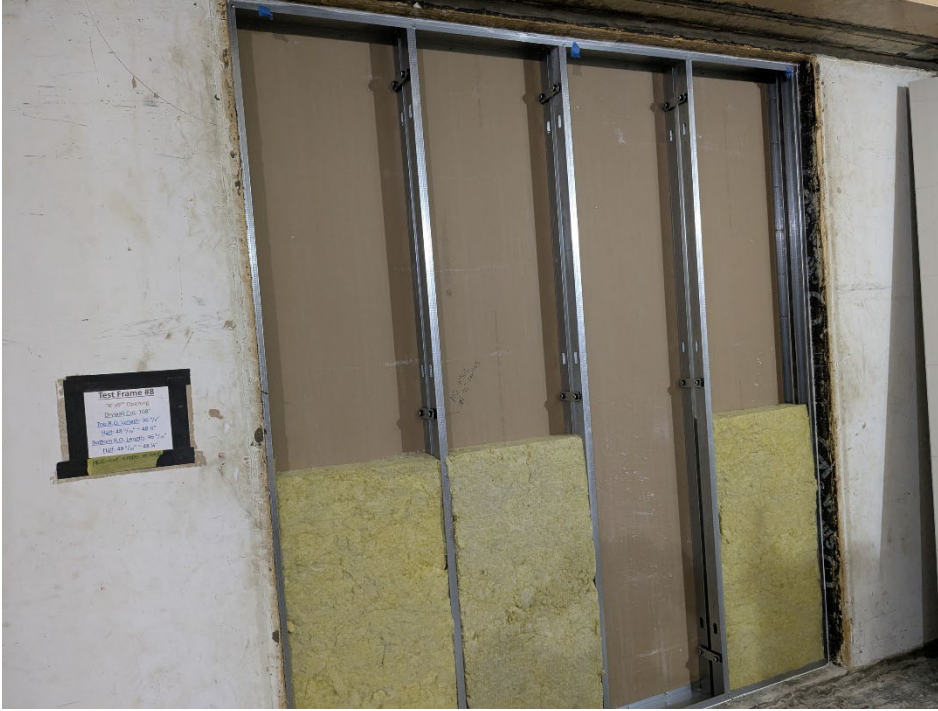
Figure 7 – Insulation partially installed in stud cavities
