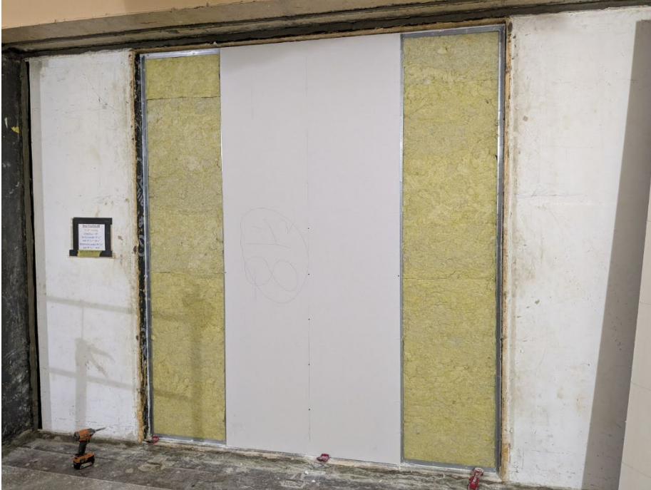
Figure 9 – Gypsum board partially installed on receive side
