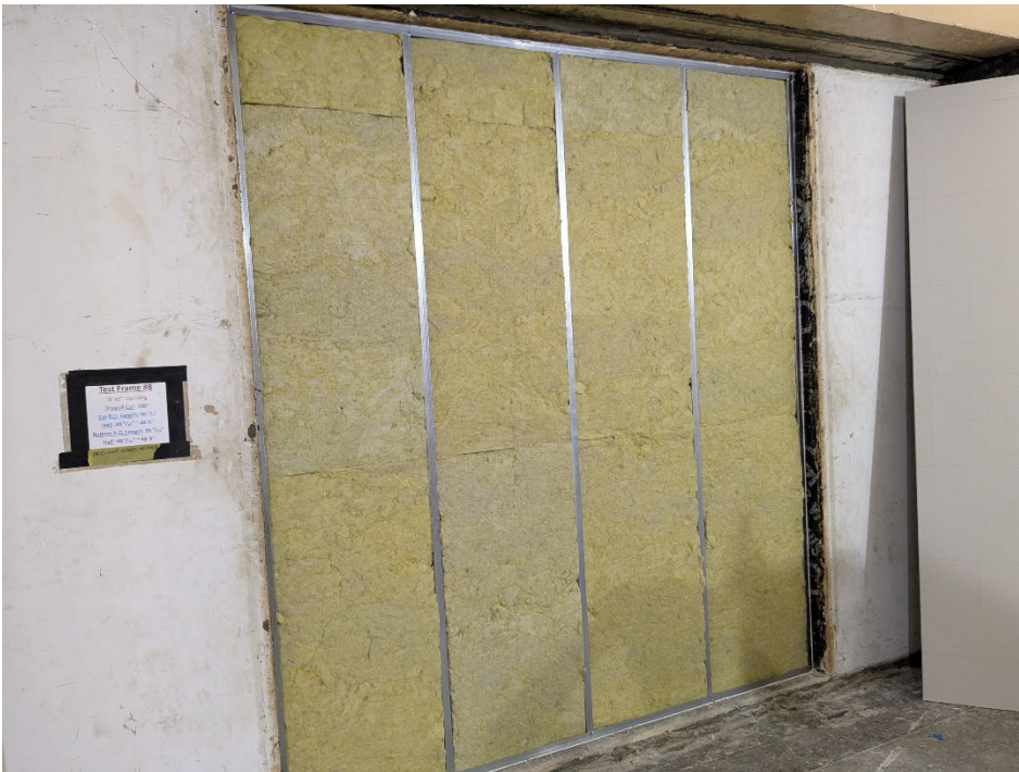
Figure 8 – Insulation installed in stud cavities
